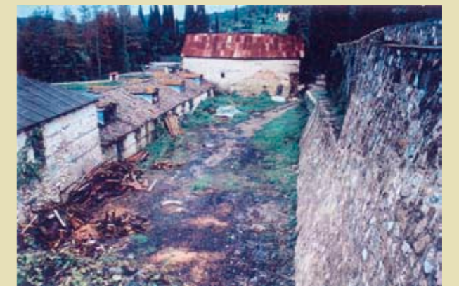
Heybarn Complex before reconstruction
