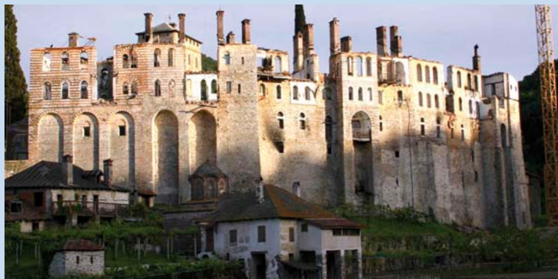
The 1816–1821 Lodge after the fire, view from the north
