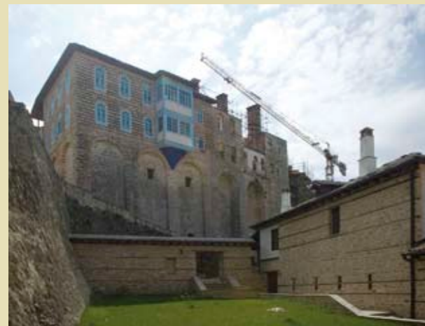
The 1814 Lodge after reconstruction, view from the Heybarn Complex
