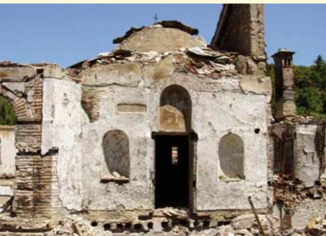
St Nicholas' Chapel, entrance, after the fire
