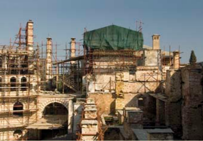
Saint Nicholas' Chapel, after the fire, view from the south
