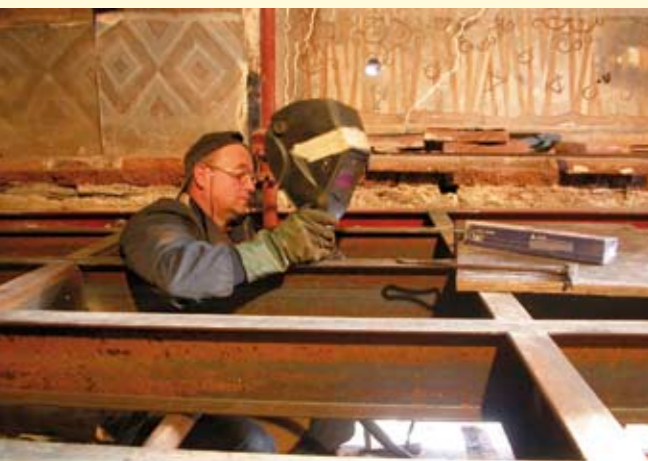
Tightening of the object with steel braces in the base area
