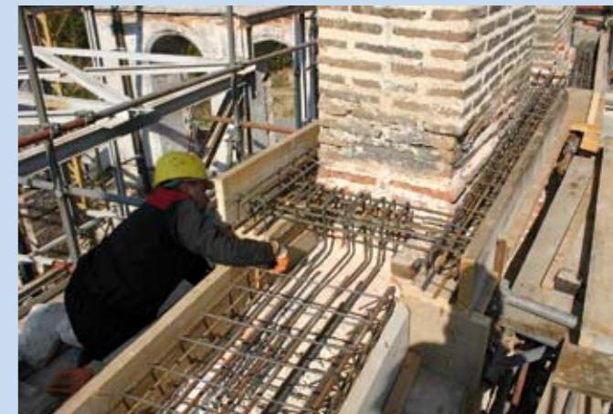
Stiffening of the walls by reinforced bond beams
