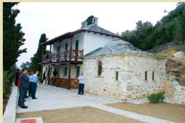
The Cell of St Stefan on Samaria Hill after reconstruction
