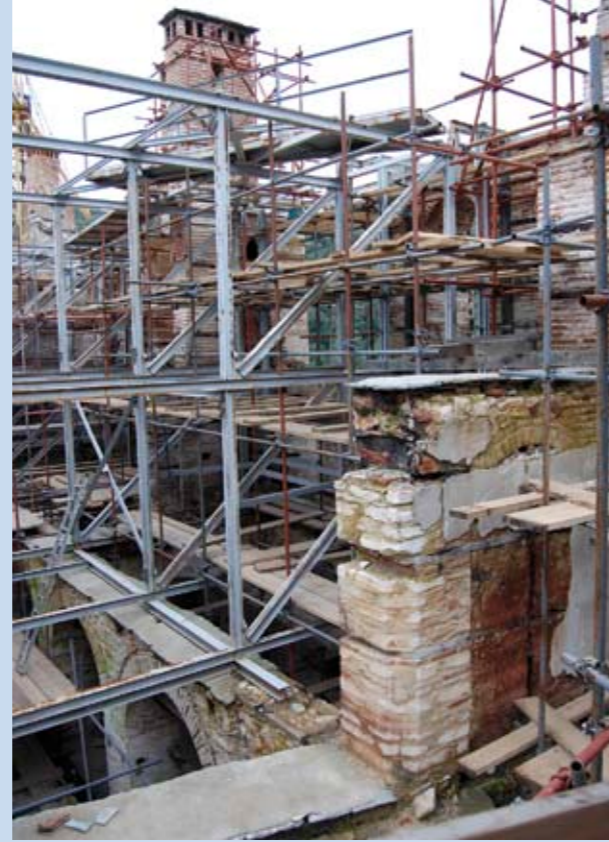
The 1816–1821 Lodge, temporary shielding structure, detail
