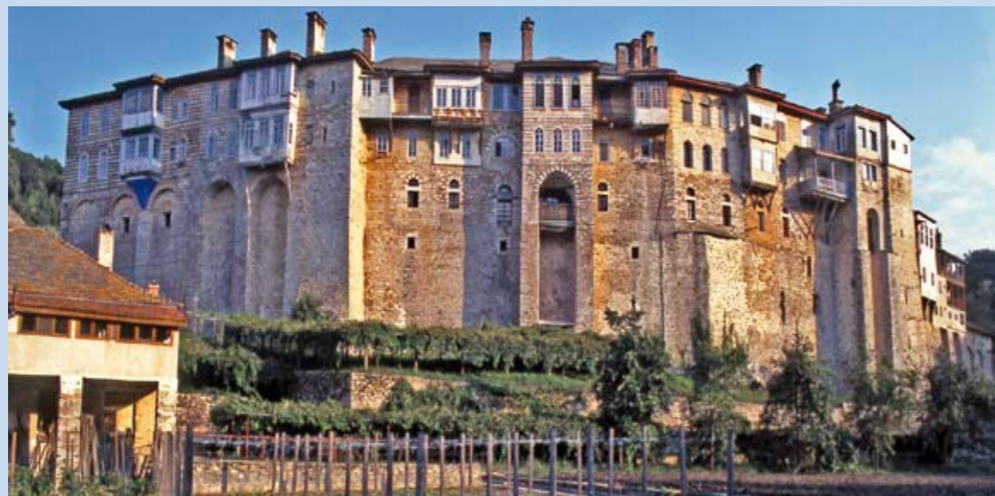
The 1816–1821 Lodge before the fire, view from the north
