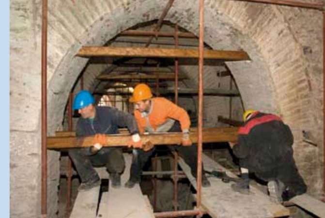
Installing of wood-coated stainless steel braces
