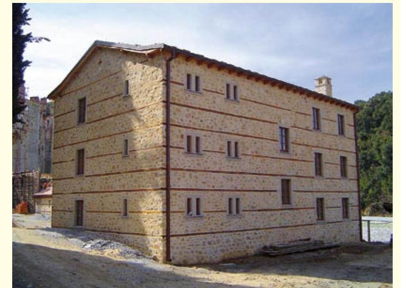
Heybarn Lodge after reconstruction
