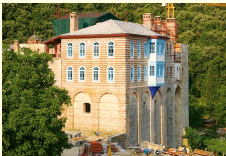
The 1814 Lodge after reconstruction
