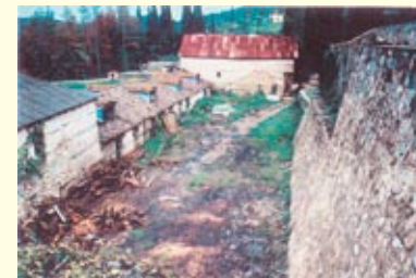
Heybarn Complex before reconstruction
