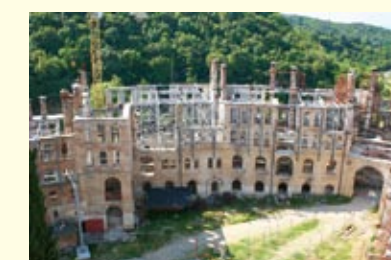
The 1816-1821 Lodge after the fire with the temporary shielding structure
