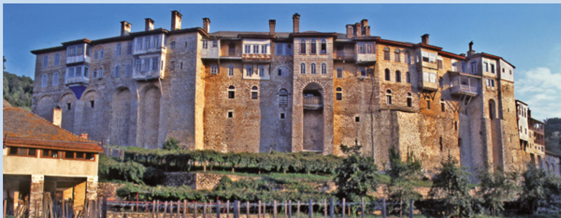
Northern part of the Monastery with the Great Residence, before and after the fire and under reconstruction
